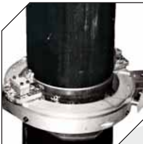
Sever the casing above the wellhead.
