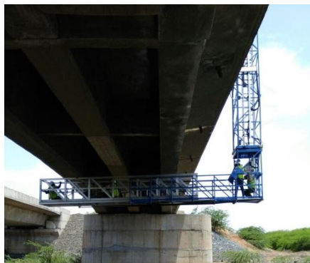
Working on a bridge near Porbandar, GJ
