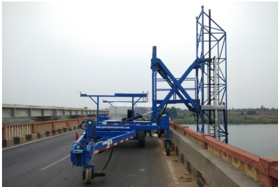
Working on Godavari Bridge Near Eluru, AP
