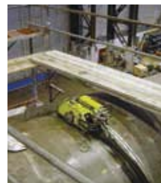
Trav-L-Cutter being used for submarine decommissioning
